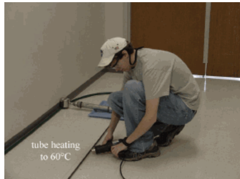
Figure 5 Tube Heating during Oligomeric Silane Cure Process
