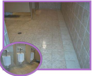
**Situation:** Potential slip & fall hazards on tile floors that are constantly wet caused the Great Wolf Water Park management to seek a system that improves coefficient of friction on all floor tile surfaces surrounding the water park experience, as well as the tile floors in the changing rooms, restrooms and shower areas. Plus, the slip mitigation system employed could not obscure the natural beauty of the tile and must remain easy to clean and maintain.
