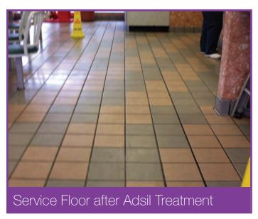
**Solution:** The Adsil MicroGuard®/MicroGrip™ Anti-Skid Floor System was applied to ceramic tile in customer service areas and on walkways in dining room areas to reduce slip & fall liability risk. MicroGuard® AD703 Clear was applied, without the MicroGrip™ Anti-Skid Additive, under tables, in bathrooms and in seating areas.
